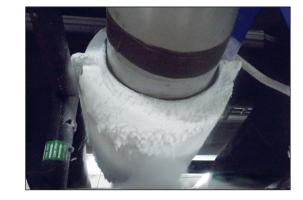
Pipe freezing is a valuable tool in the maintenance of all types of liquid storage, process and transfer plant.
